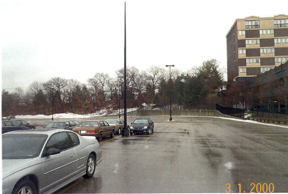
Southwest corner of site looking at Holiday Inn/retaining wall
