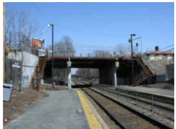
Existing Morton Street Station
