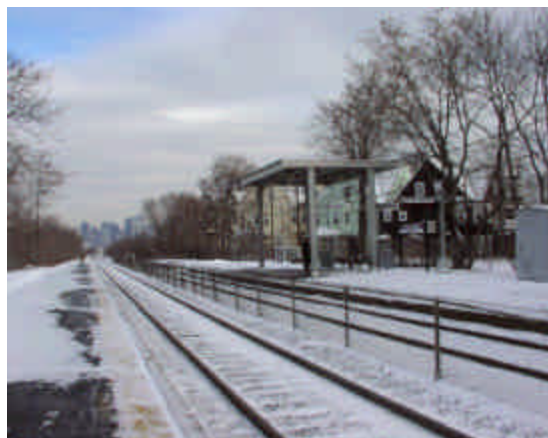
Existing Uphams Corner Station
